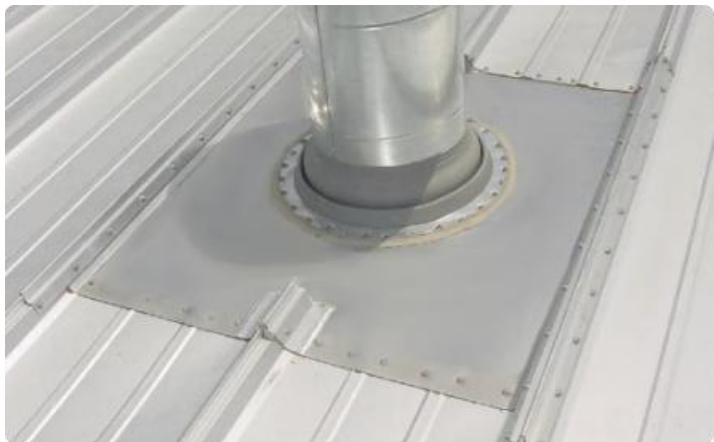
Roof Flashing
